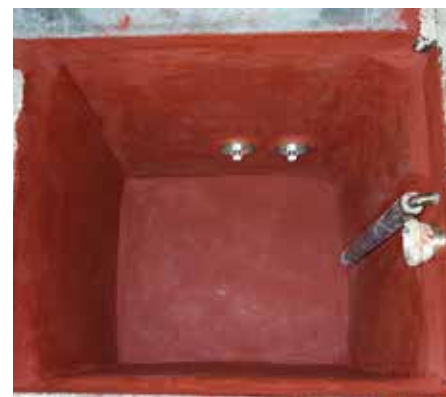
Sump after coating
